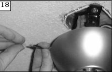
Make wire connections to power source using wire nuts provided. Make sure that no filiments are outside of the wirenut. After making the wire connections, the wires should be spread apart with the grounded conductor and the equipment-grounding conductor on one side of the outlet box and ungrounded conductor on the other side of the outlet box.
